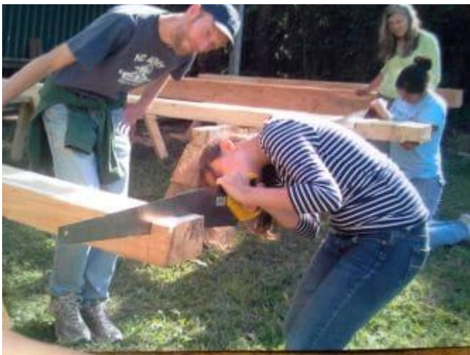
Kenna, in the green shirt, along with MFS students and staff, learn timber framing to build our amazing meeting room.
