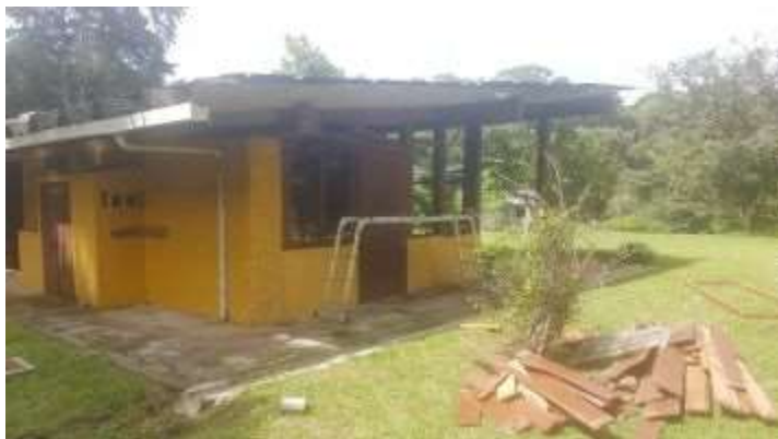
An outdoor view of the side of Puffers and a picture of the structure with sides torn down to the cement part and steel window beams added.
