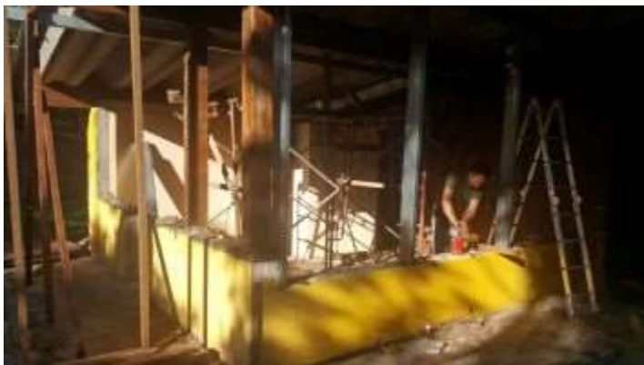
An outdoor view of the side of Puffers and a picture of the structure with sides torn down to the cement part and steel window beams added.
